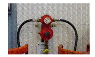
• All regulators that are not connected directly to a cylinder i.e. those connected by a hose, should be positioned above the top of the cylinder
